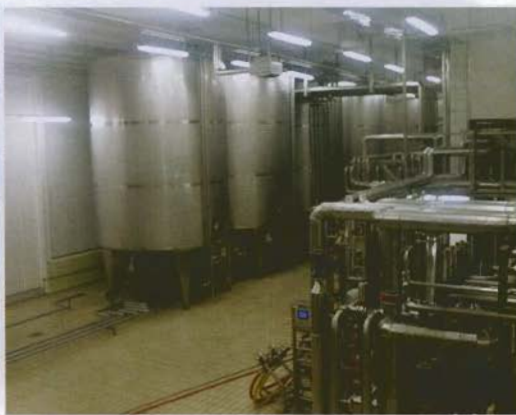
View into the basement of the new production building in Ljubljana
